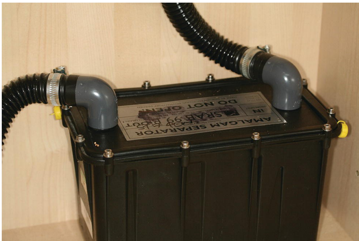
Figure 15.27 Waste amalgam separator trap under sink.
