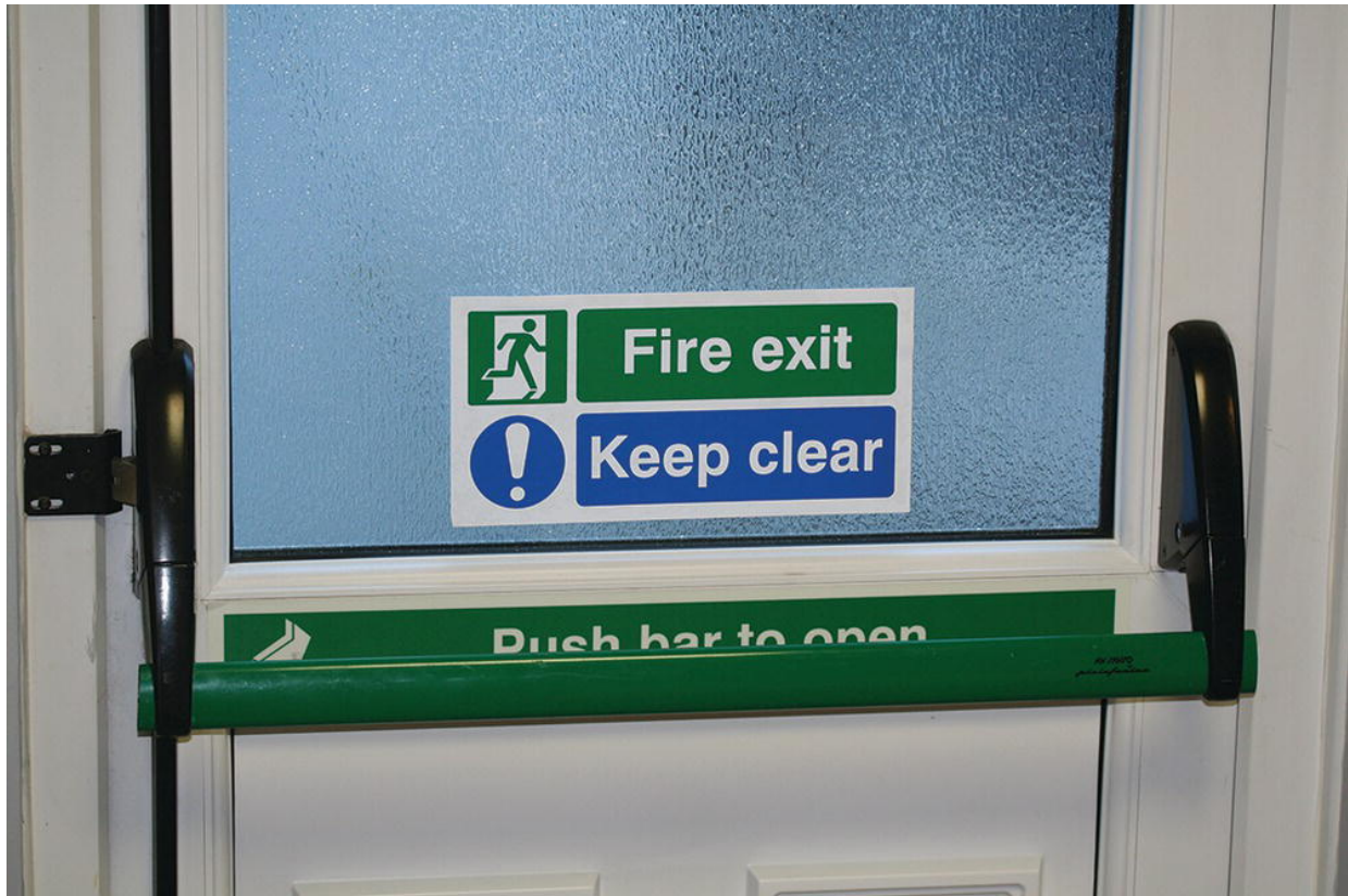
Figure 4.29 Push-bar operated emergency fire door.
